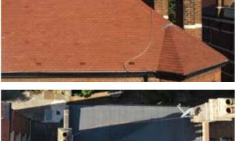
The small flat roof has been constructed with an overlapping felt system which appears to be in a good condition. The overlaps are in good condition with no sign of coming away. There is no staining or vegetation on the roof.
